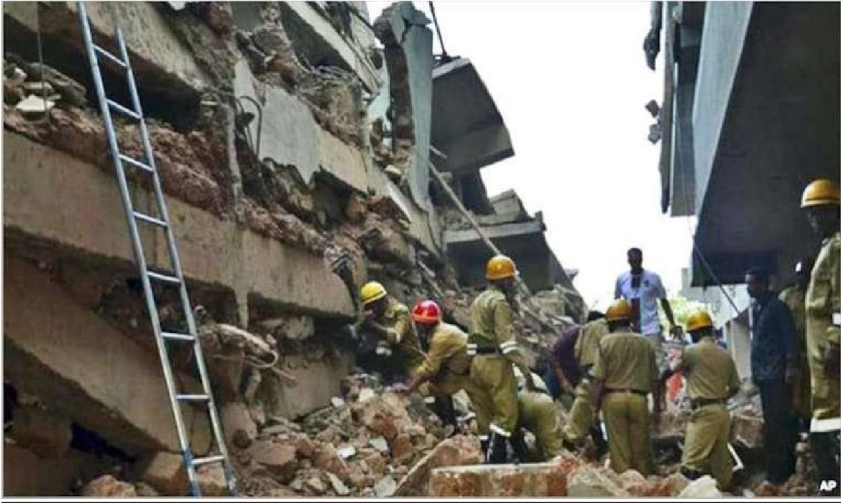
Fig 1: Rescue team reached the site after collapse
