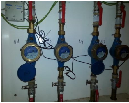
FIGURE 3.4: M-BUS, SECONDARY WATER METERS AT LOCATION VRBANI III, KUTNJAČKI PUT 10
