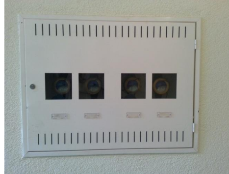
FIGURE 3.4: M-BUS, SECONDARY WATER METERS AT LOCATION VRBANI III, KUTNJAČKI PUT 10
