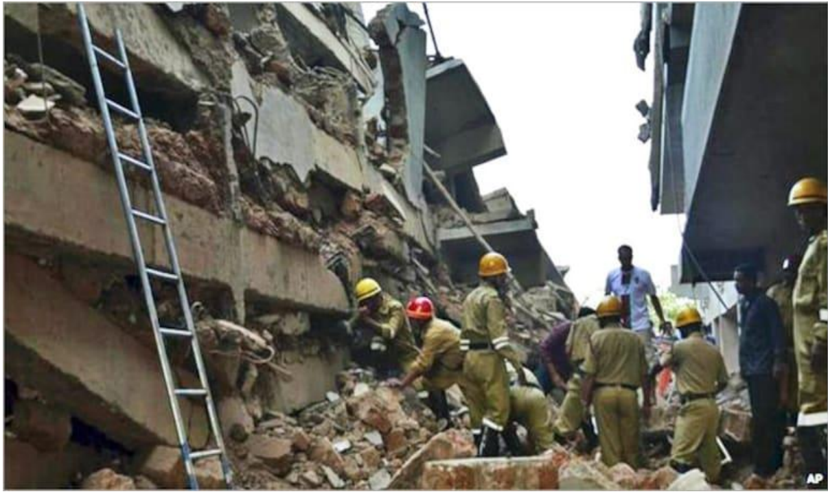
Fig 1: Rescue team reached the site after collapse
