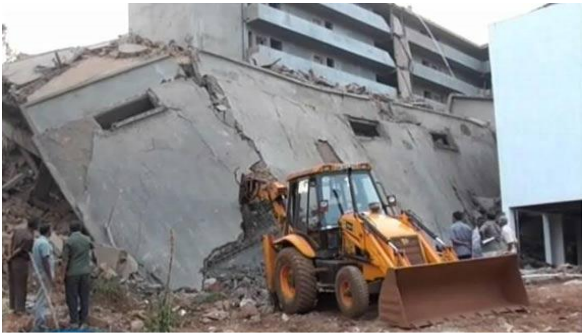
Fig 3 : Crane trying to remove debris from the area
