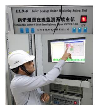
Figure 24 Author Inspecting the Boiler Tube Leak Detection System
