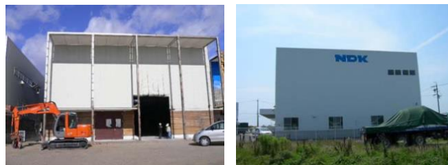
Fig 1.4. Left: Qatar pavilion after EXPO 2005, Right: Nippon Denshi Kogyo Source: Expo 2005
